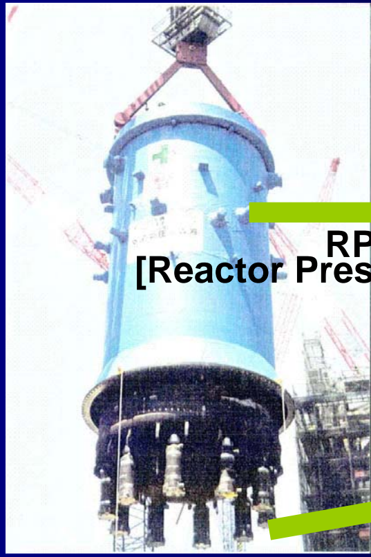
RIP [Reactor Internal Pump]
